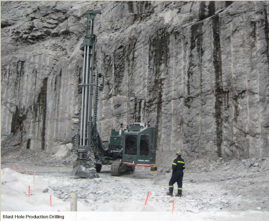
Blast Hole Production Drilling
